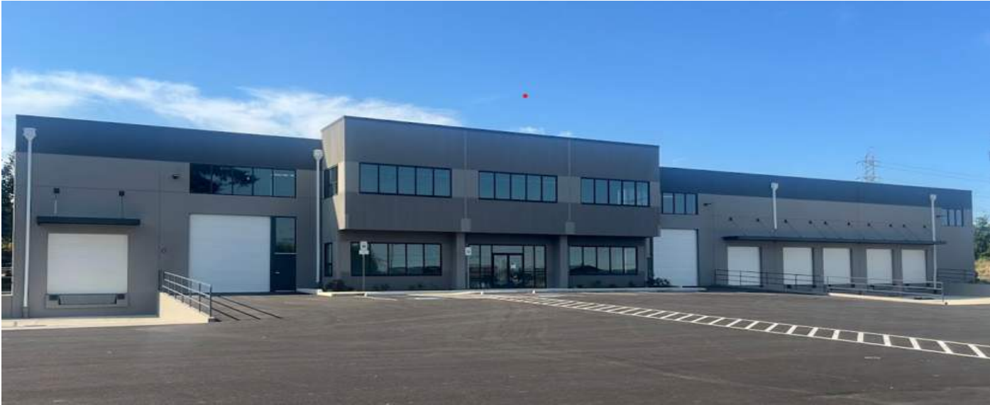
BARKER BUILDING #1 (EXISTING)
