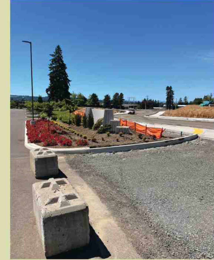
Ice Age Drive under construction
