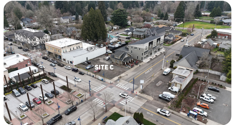
Fig. 20. Site C- BEFORE
