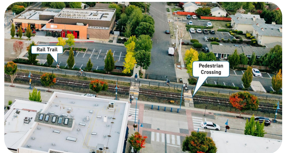
Fig. 17. Washington Street w/Rail Crossing - AFTER
