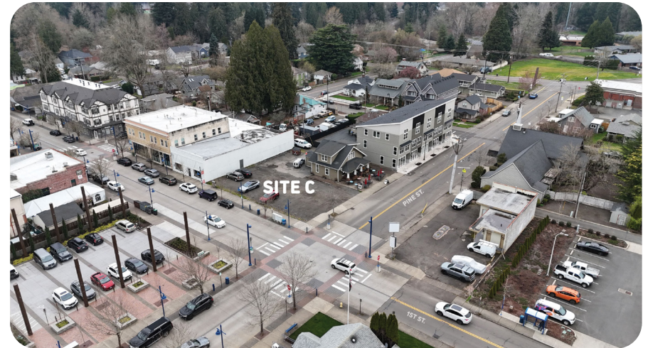
Fig. 20. Site C- BEFORE
