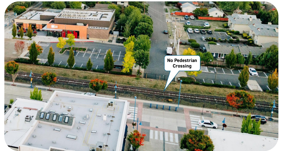
Fig. 16. Washington Street w/No Rail Crossing - BEFORE
