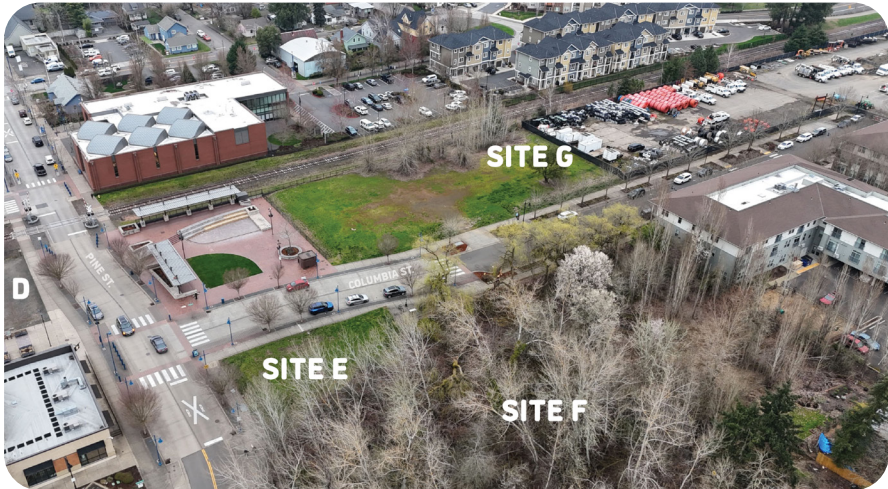
Fig. 24. Site G- BEFORE
