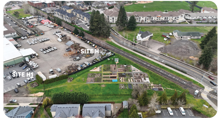
Fig. 26. Site H & H1- AFTER
