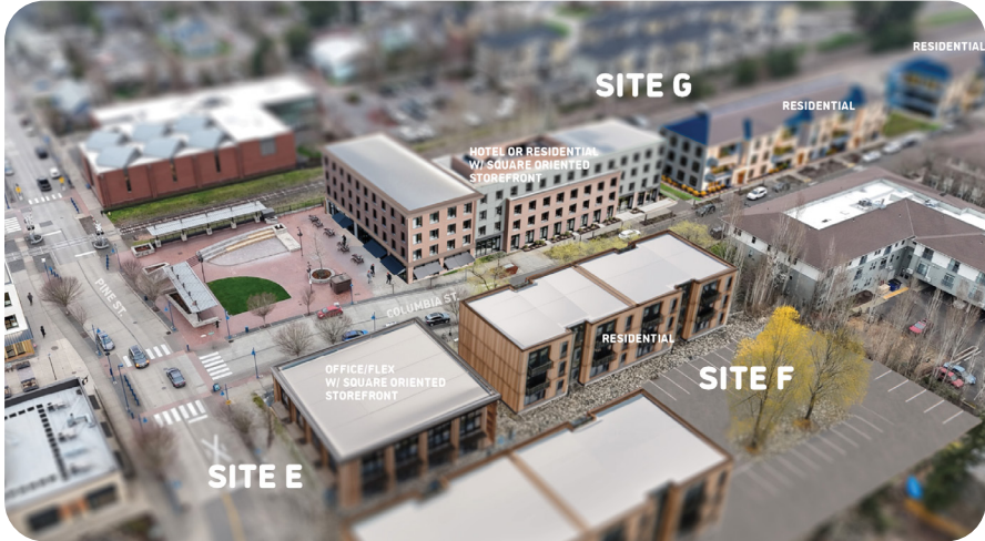
Fig. 25. Site G- AFTER
