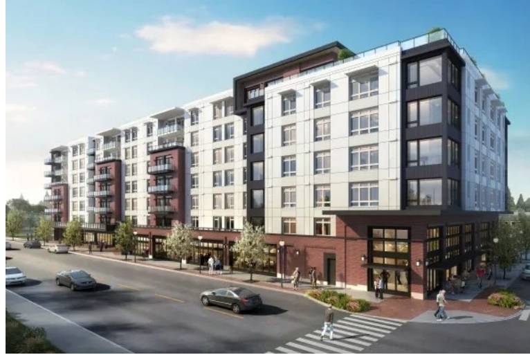
Merrill Gardens at Hillsboro 146 NE 4 th Avenue Hillsboro, OR
