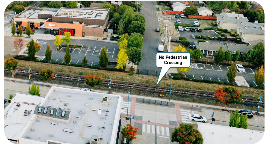
Fig. 16. Washington Street w/No Rail Crossing - BEFORE
