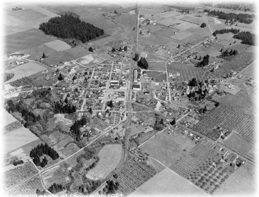
Aerial photo of Sherwood, 1951
