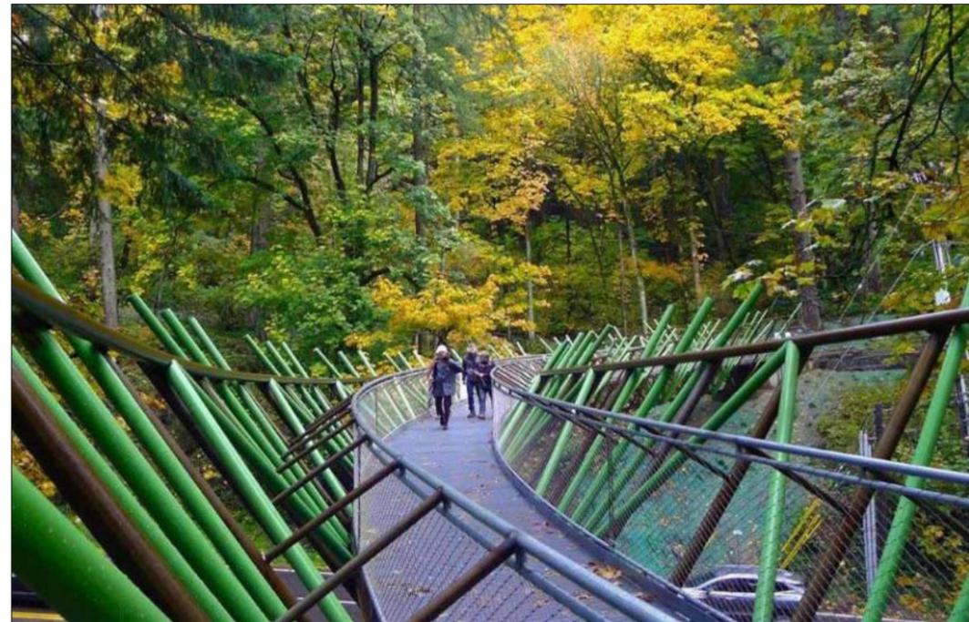
**Curved Triangular Section Truss**
