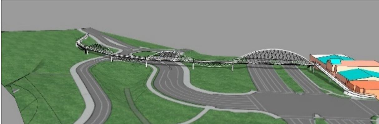
In this approach, the inherent material efficiency and cost effectiveness of a tall arch form is exploited across the length of the entire structure. The net effect is the appearance of a single, undulating structure that increases in arch size from the west, culminating in the primary span across Hwy 99W.
