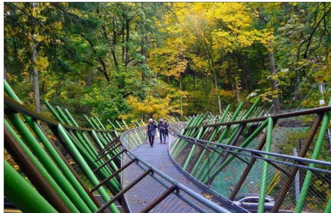
**Curved Triangular Section Truss**
