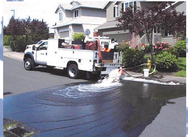
Most of the time fire hydrants are used to flow between 1300-1600 gpm to scour the mainlines. The duration of the flushing is based on the size of pipe, the length of pipe, the field turbidity/chlorine measurements and the goal of 1 exchange of water in the pipe being flushed. In addition to removing sediment in our water pipes staff is able to confirm proper operation of valves and fire hydrants. All water is de-chlorinated prior to entering the storm system.
