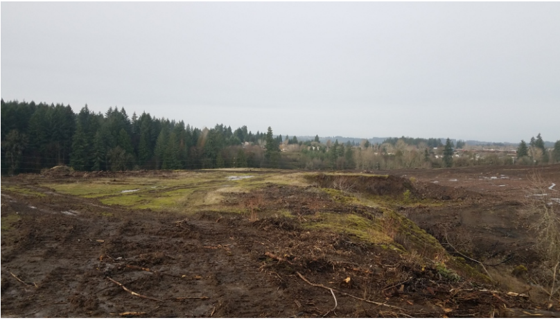
Photo 1: TL 100 view west along rock pit. Imagery date: December 2018
