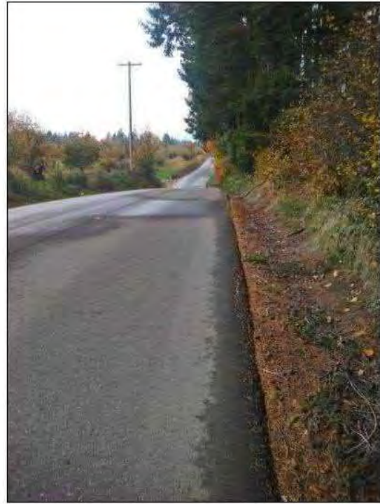
B. Main Site Access Looking West
