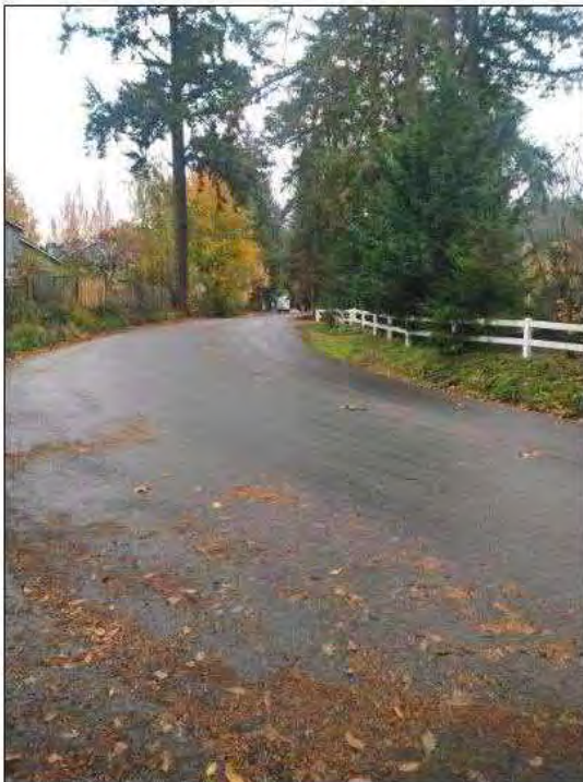
C. Shared Driveway Looking East
