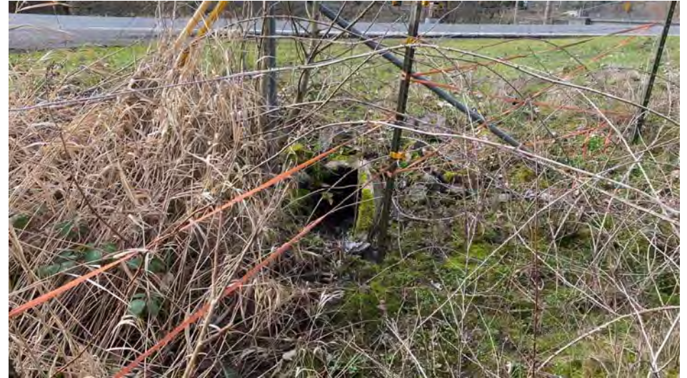
Photo J. View of culvert under SW Tonquin Road within Wetland A.
