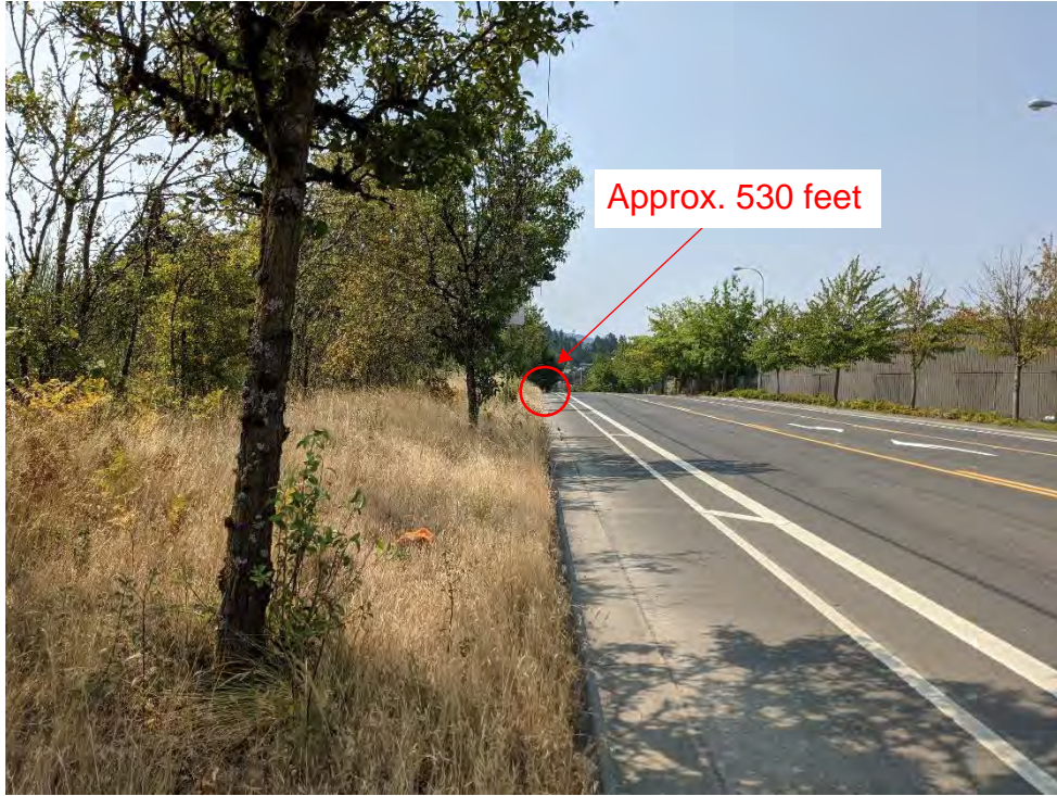
Figure J3. North Access Looking Left, Car
