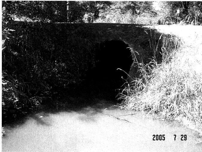
Washington Street Culvert
