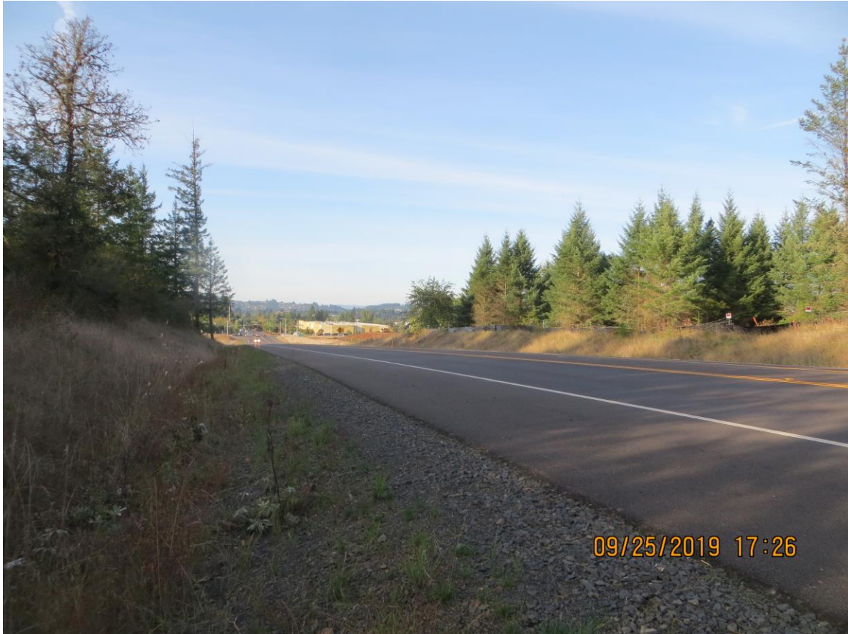
Figure 6. SW 124 th Ave/SW Blake St looking south
