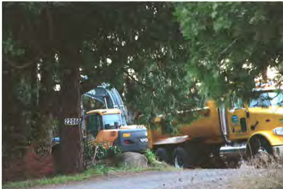
Figure 4 Example of Construction Equipment being used and stored on TL #2100
