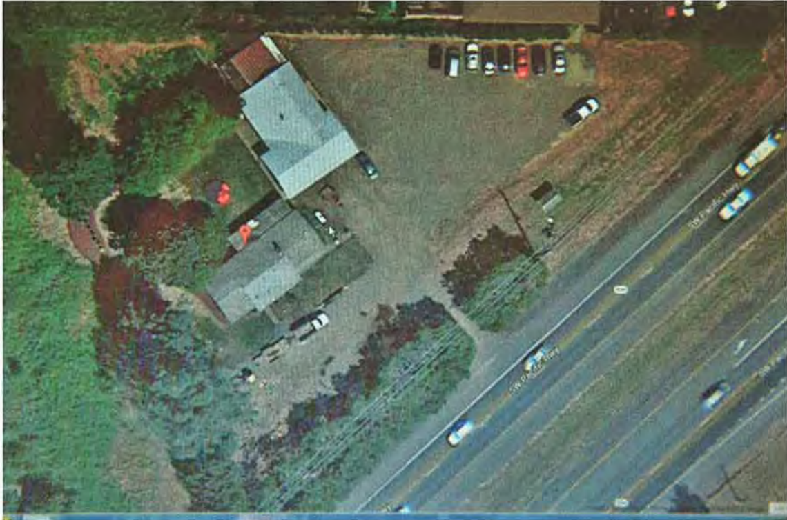
Figure 3 Aerial View of TL #2100 after Illegal Conversion to Parking areas and removal of trees
