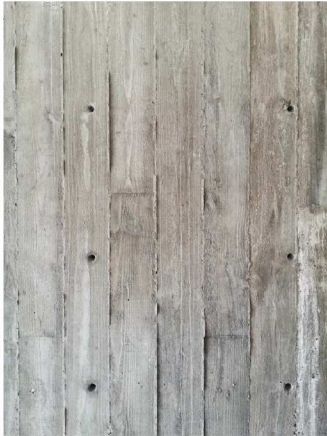
CONCRETE: BOARD FORMED
