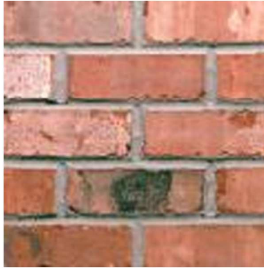
MUTUAL USED BUILDING 'A'
