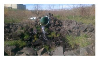
Figure 6. Outfall piped across floodplain to Rock Creek
