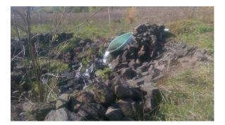
Figure 1. Outfall piped to the edge of Rock Creek
