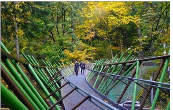
**Curved Triangular Section Truss**
