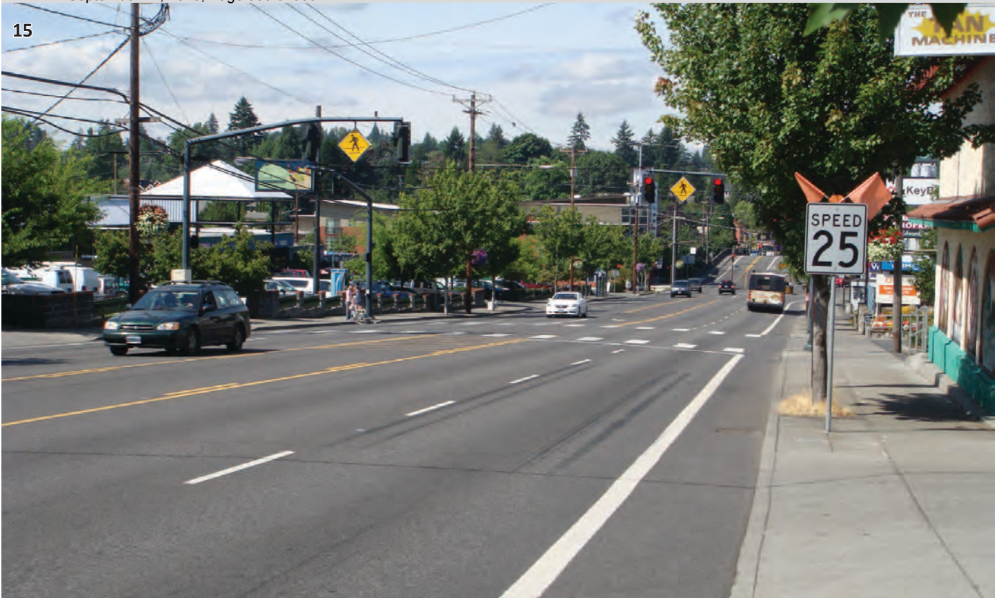
Image 15: High-visibility crosswalks, bicycle lanes, and a road diet to five lanes could make Highway 99W safer and more pedestrian friendly.
