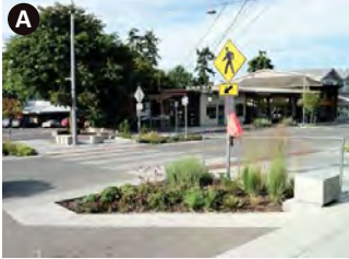
"Complete Streets" along 99W, Sherwood Blvd., and in Old Town support calm roadways safe for all users, stormwater and landscape features, attractive streetscapes, and easy access for people on foot and bicycle.
