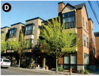
Medium intensity mixed-use commercial and residential in Old Town in Alternative 3 provides employment and living options that blends with Old Town's character.
