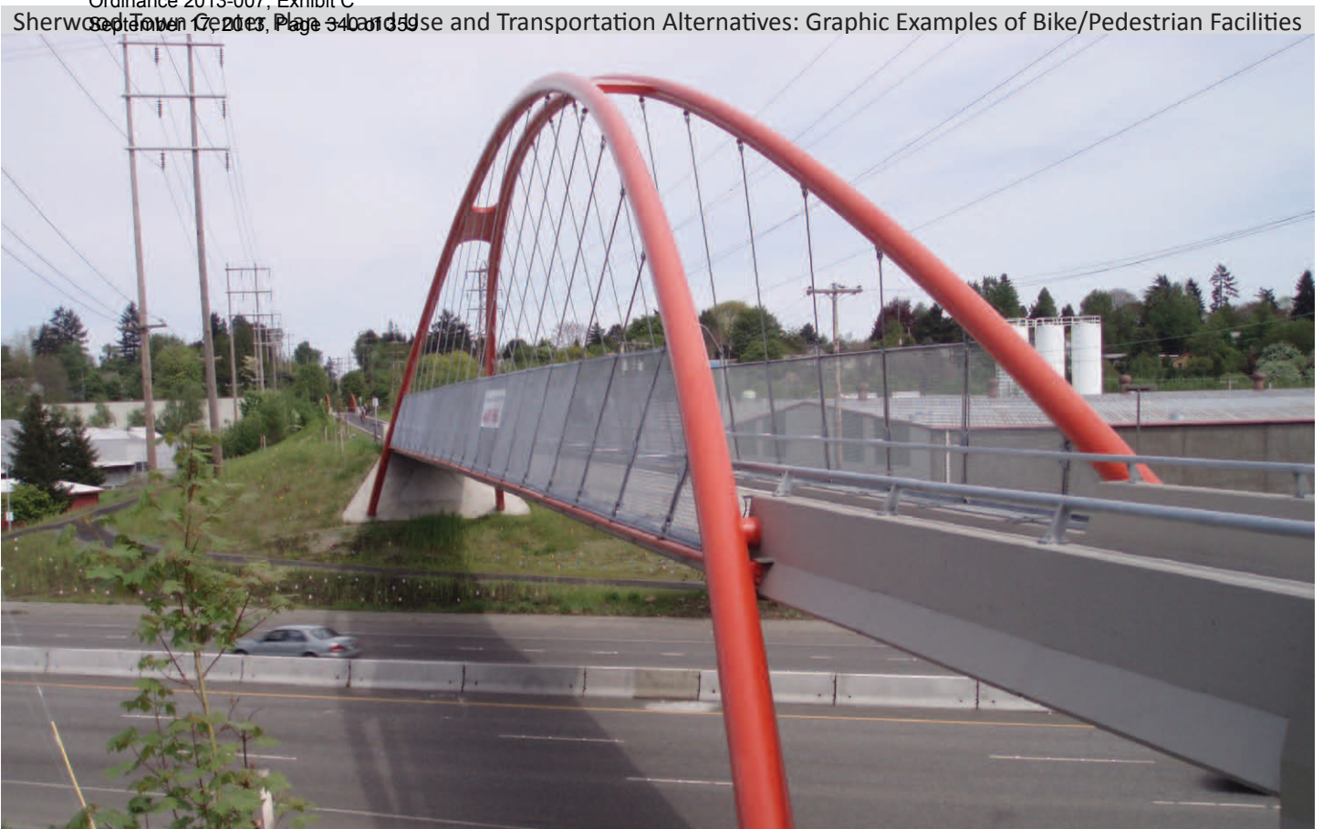
Image 5: Grade-separated bicycle/pedestrian crossings represent one option for reducing the Highway 99W barrier effect.
