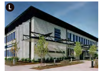
Medium-scale light industrial and office uses around Tualatin-Sherwood Rd. bolster the employment base in Sherwood.
