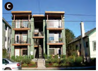
Medium-scale multi-family residential can coexist next to single-family detached homes in well-connected neighborhoods around Old Town.*
