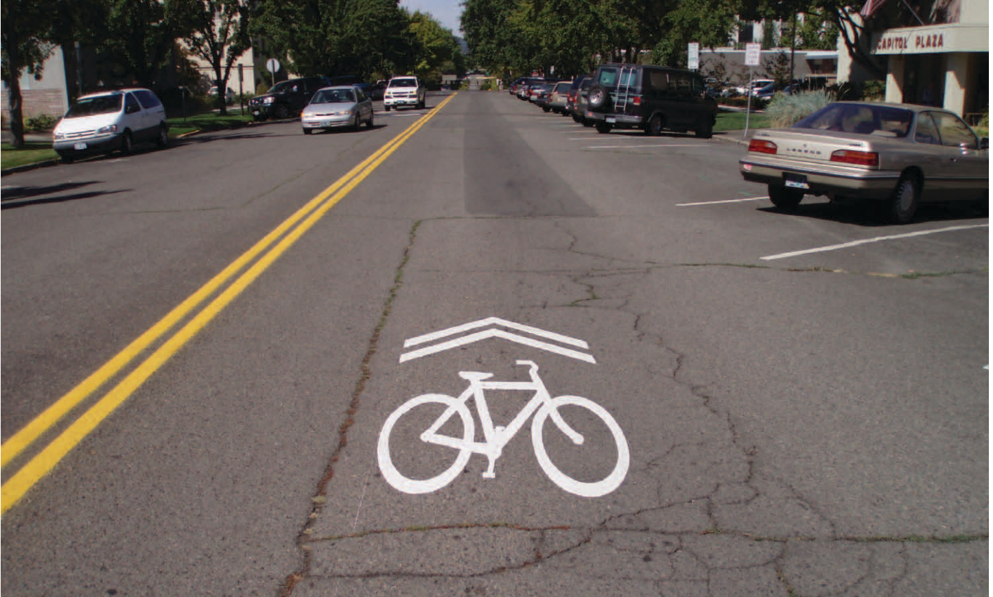
Image 1: Shared lane markings can heighten the visibility of people on bicycles in areas where cyclists and motorists must share the roadway.
