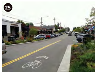
Old Town streets can be given a "Complete Street" treatment (where currently lacking) with on-street parking, wide sidewalks, stormwater facilities, and shared roadways for autos and bicycles.
