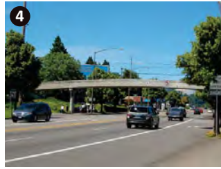
In the long-term, a grade-separated crossing of Highway 99W can reduce the "barrier" effect of this large roadway.
