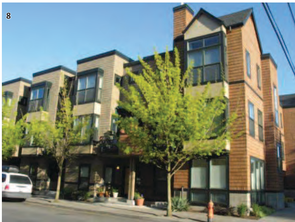
Image 8: Three-story apartments can increase residential density.
