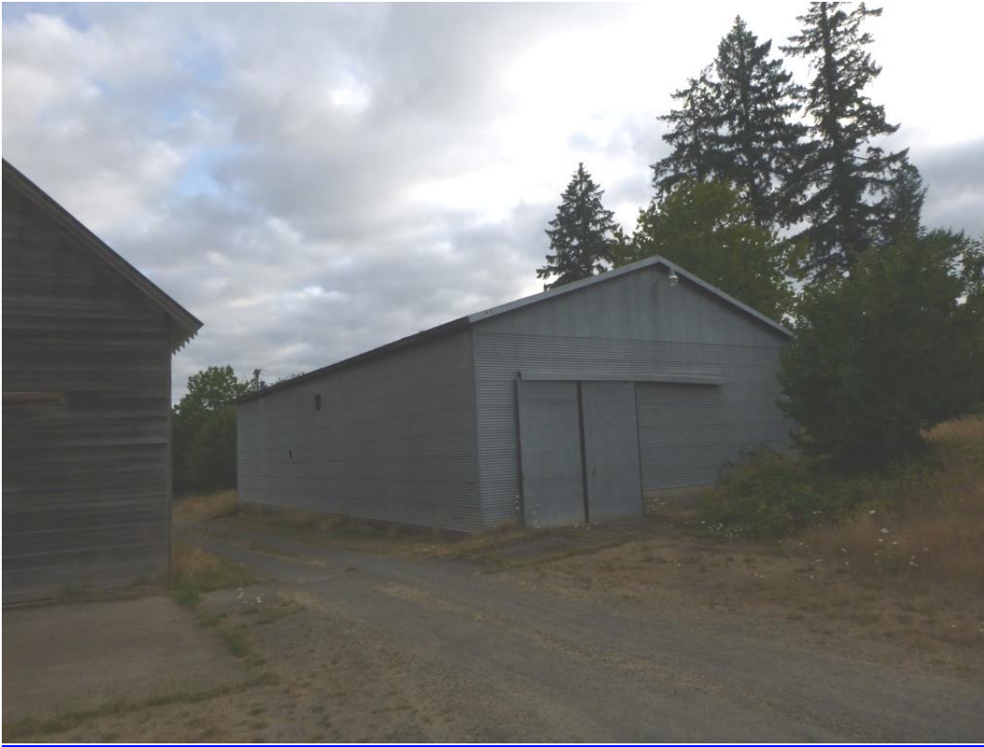
Outbuilding 1 at 20555 SW Gerda Ln. (ca. 1970); view northeast.
