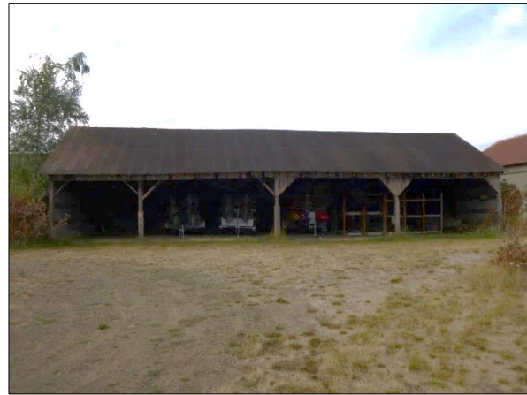
Figure 5.2.1-5. Three-sided barn at 20555 SW Gerda Lane (ca. 1952); view south.
