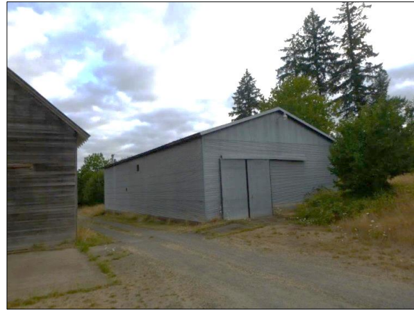
Figure 5.2.1-3. Outbuilding at 20555 SW Gerda Lane (ca. 1970); view northeast.
