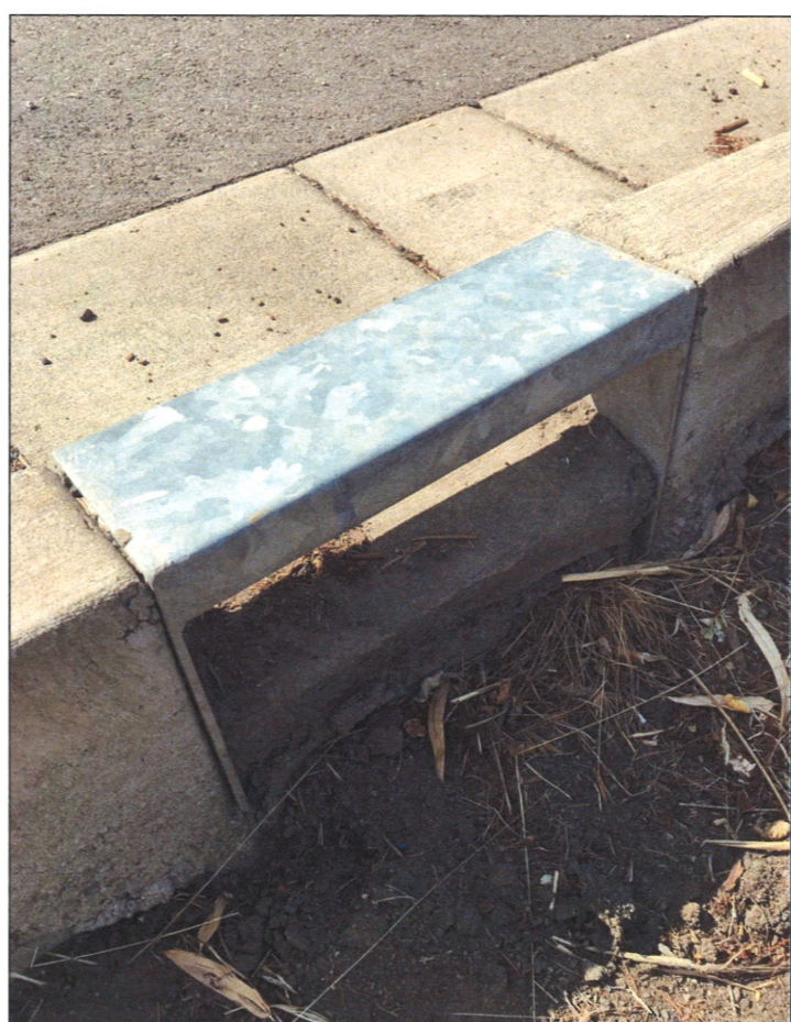
SAMPLE CURB OPENING CURB OPENING TO BE MADE OF GALVANIZED STEEL WITH 18" OPENING AND 2" DEEP TOP PLATE COVER. GET SUBMITTAL TO INSPECTOR FOR APPROVAL PRIOR TO PURCHASE.
