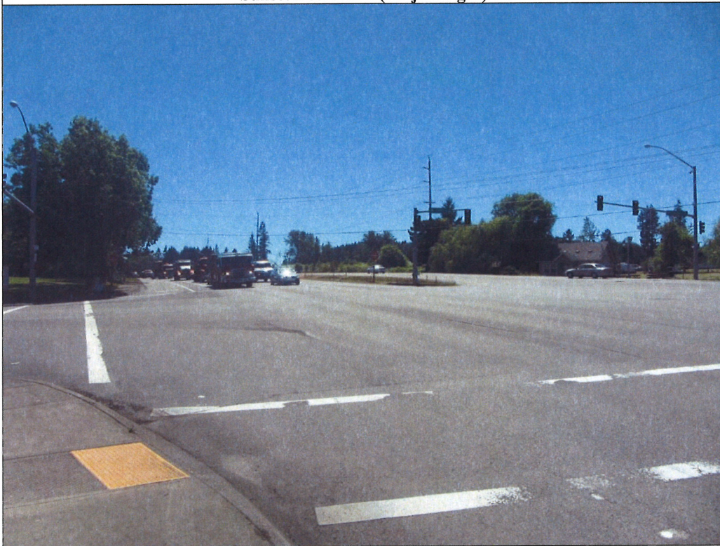
Westerly street scene along Southwest Pacific Highway overlooking its intersection with Sunset Boulevard
