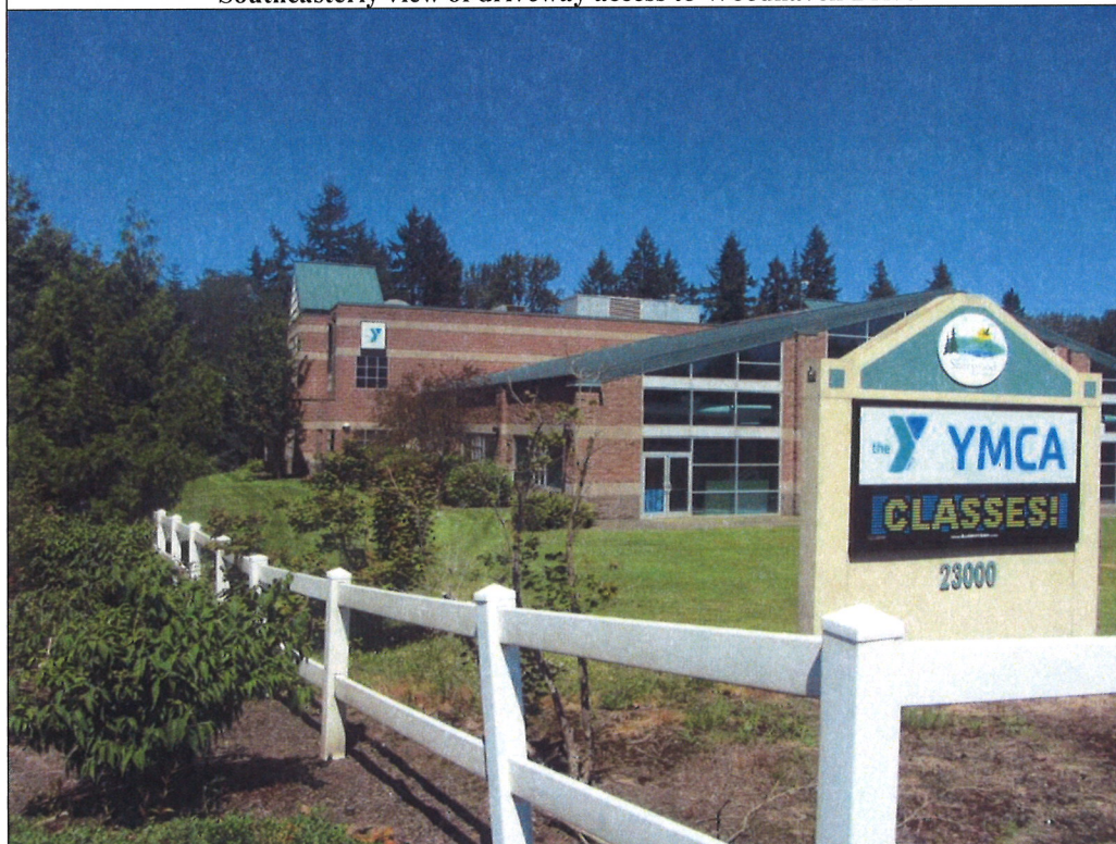
Northeasterly rear view of subject property
